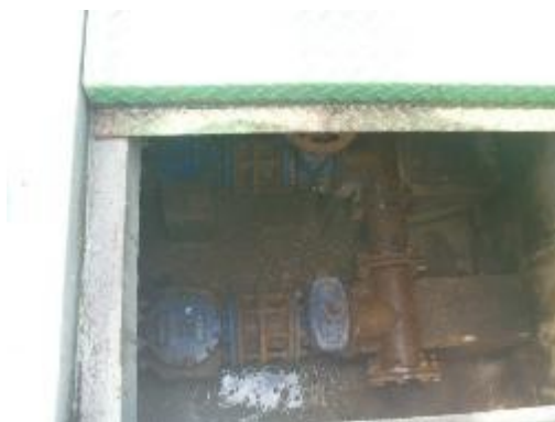
Barrilete de recalque
