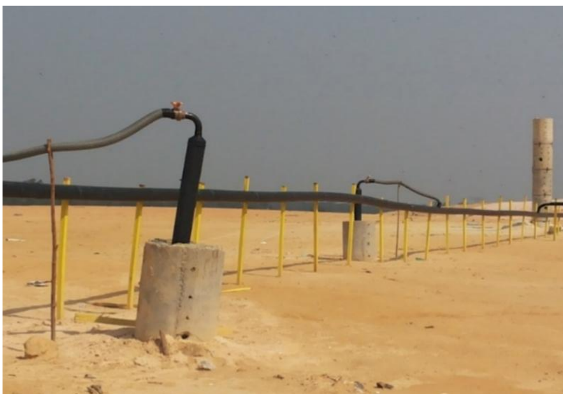
Figura 80 – Dreno vertical de gases
